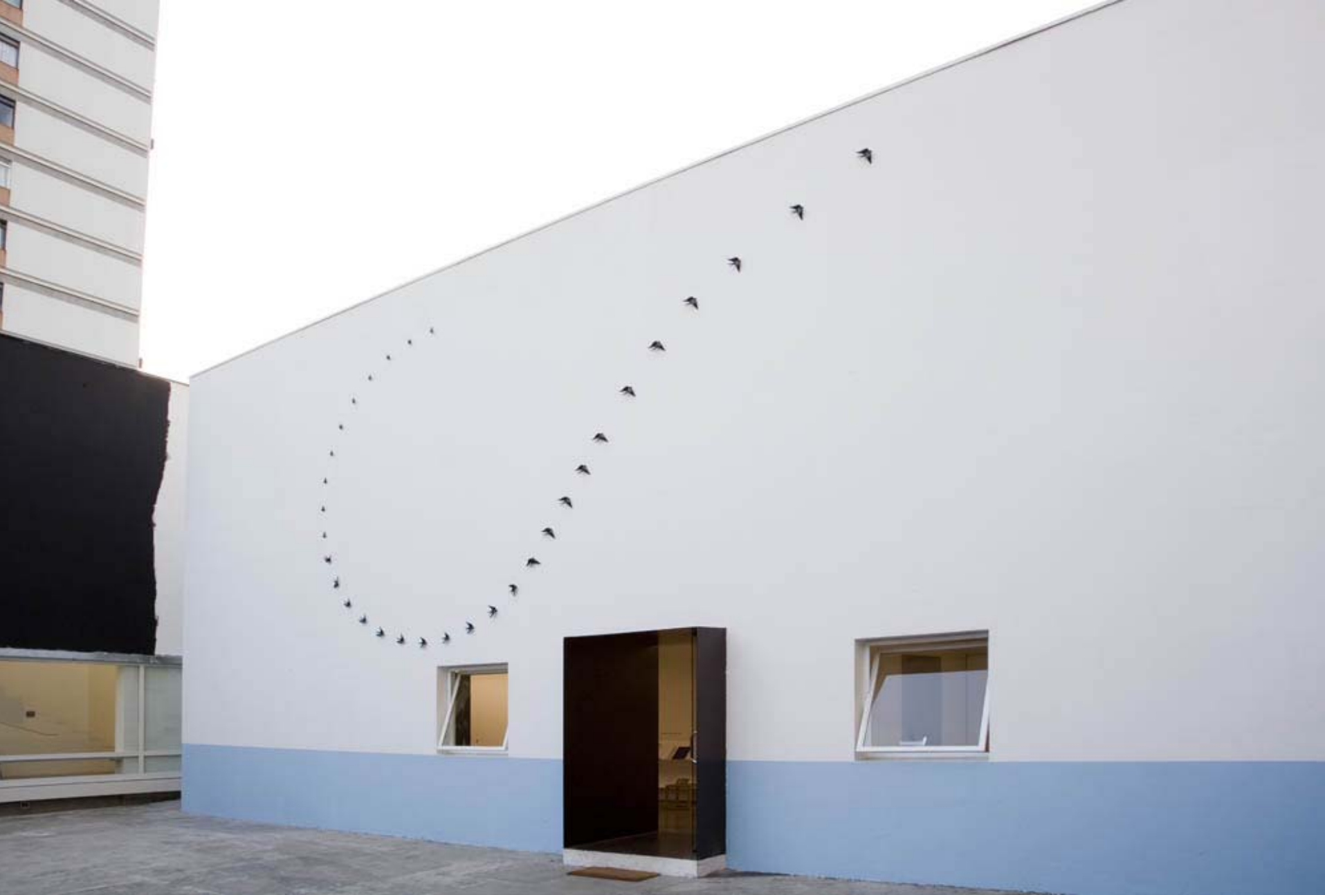
Fachada/ facade Andorinhas (2007) – Gabriela Albergaria
